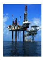
The offshore oil industry long ago chose the jack-up as the platform-of-choice to support the heaviest loads in the harshest ocean environments in the world. The jack-up has been known to carry loads that are far greater than any of today's largest offshore wind turbines. Its unique design elevates the entire substructure well above the waves reducing many of the hydrodynamic loads that wreck havoc on conventional wind turbine foundations.
